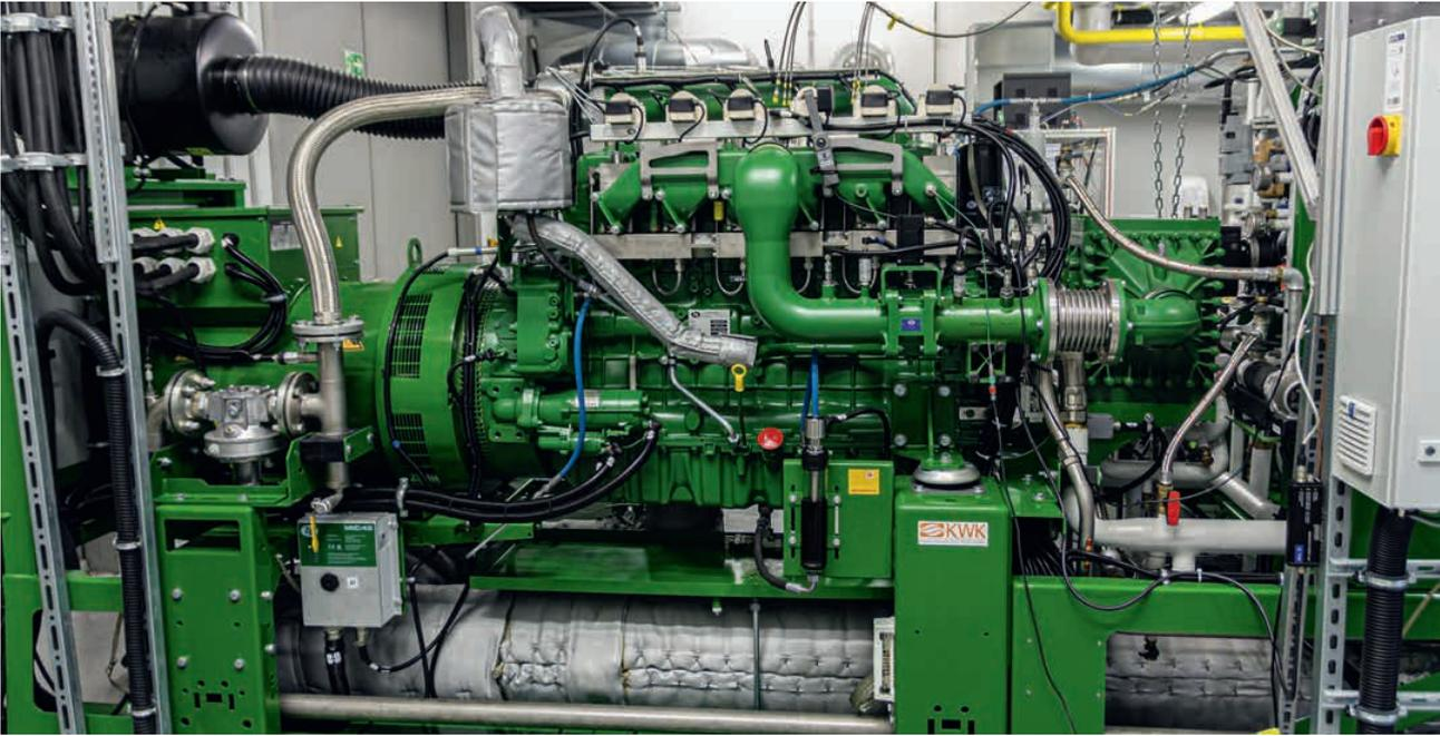
The converted decentral CHP with added hydrogen supply
