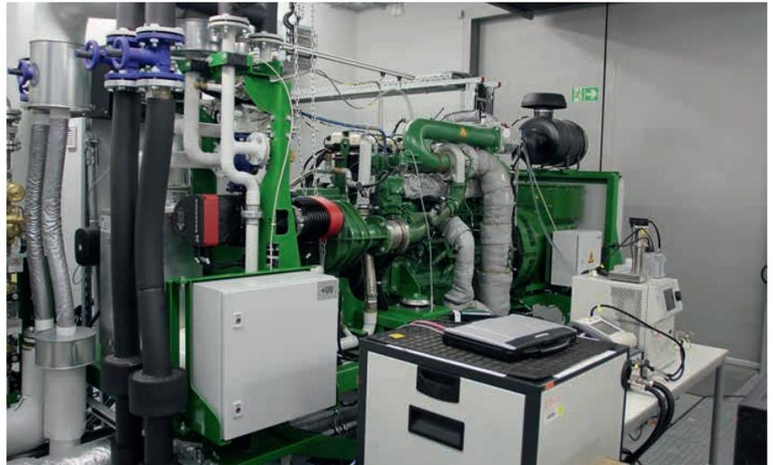
Figure 1. H<sub>2</sub> CHP plant equipped with measurement technology for combustion and emissions analysis
