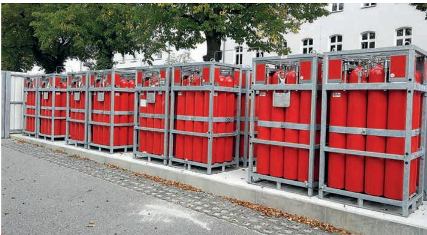
Figure 2. The hydrogen is currently still delivered in cylinder bundles
